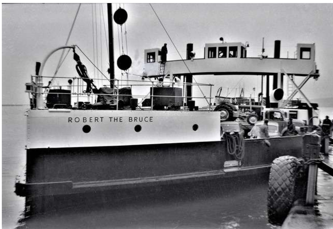
Firth of Forth car ferry " Robert The Bruce " at South Queensferry in 1960. Completed in January 1934 by Denny Brothers, Dumbarton. Double ended with a rudder at each end she was a diesel electric paddle boat of 217 GRT, her engine supplied by Paxman of Colchester. Her sister also built by Denny was of riveted construction but the above was the first ship to be completely electrically welded. Both ferries cost £22,000 to build. Made redundant by the opening of the Forth road bridge in 1964 she was sold for demolition to P. & W. MacLellan, Bo'ness in April 1965. (Photo by Martyn Hunt)
