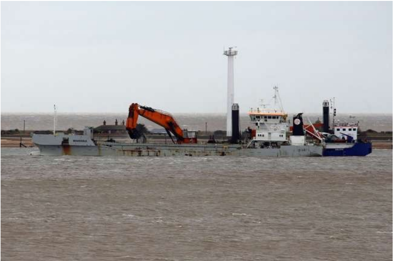
Caught in the act backhoe dredger "Goliath" deposits another bucketful of spoil into hopper barge "Boussole" on 7 th April.
