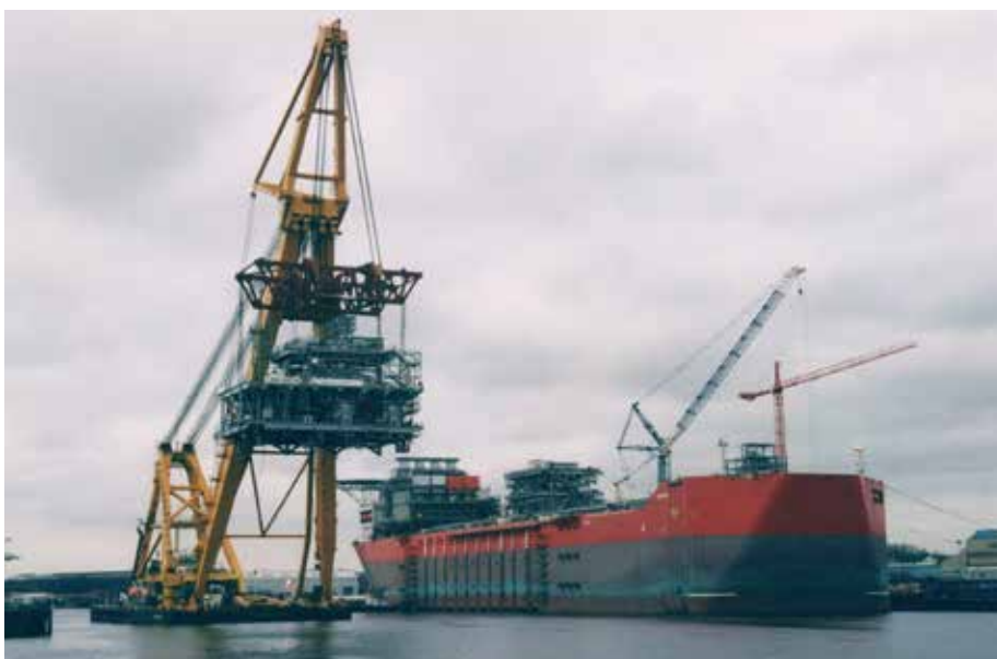
ASIAN HERCULES II lifting a module for installation on BONGA
