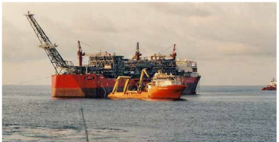
Installation work in the Bonga Field
