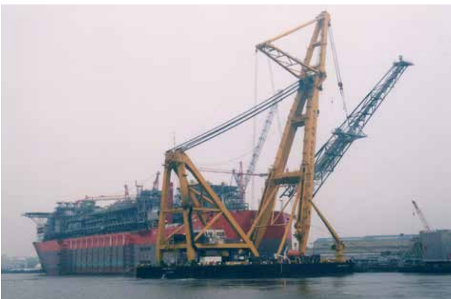
Installing the flare boom on BONGA
