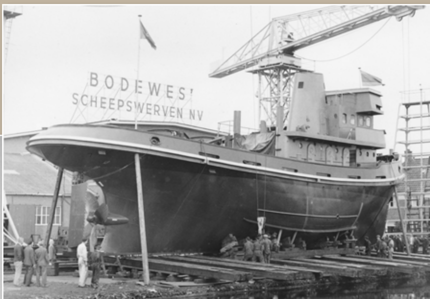
At Bodewes Martenshoek preparations are under way for the launch of EL KARIM. This 1.300 bhp tug is under construction for Société Chérifienne de Remorquage et d'Assistance, Casablanca, Morocco, for delivery in 1963. Dimensions are 29,10 / 26,30 x 7,73 (oa) x 3,81m. Draft 3,42 m. Speed 10,5 knots
