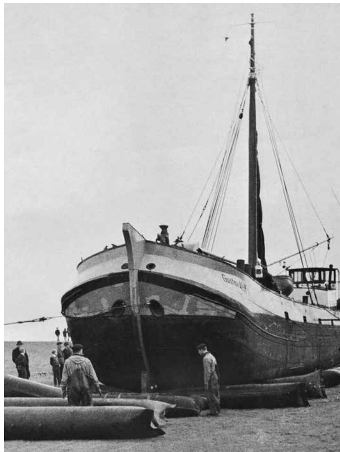
Horizontal transport over land using the “Flexodam containers”
