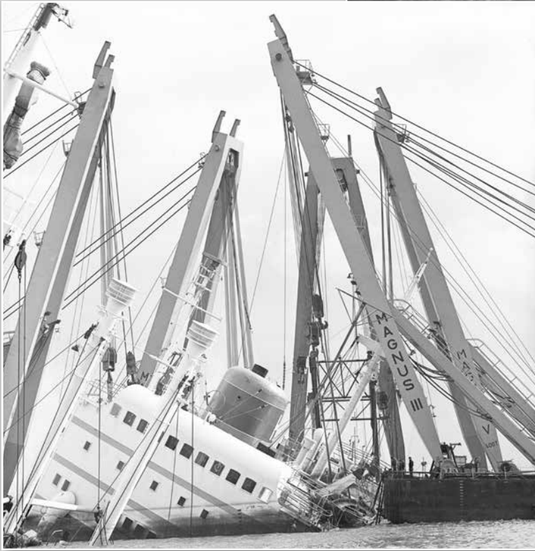
Five Harms shearlegs attempting to righten the freighter photo: Rotterdam City Archives / Ary Groeneveld (licensed under CC-0)
