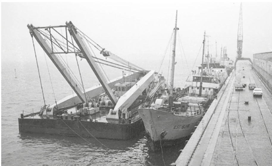
MAGNUS II at Kiel with shearlegs frame lowered in position for sea transport
