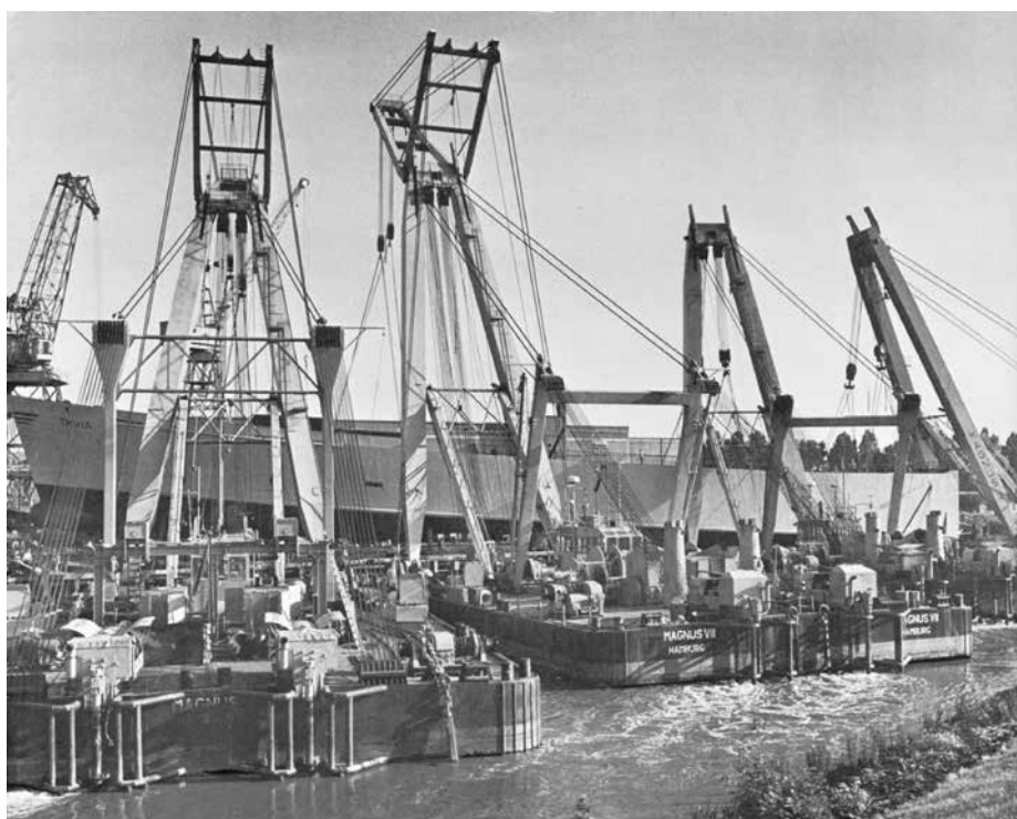
Four Harms sheerlegs effecting the launch of the 1.300 tonnes hull of THULE. Note position of deck-mounted Schottel Navigator azimuthing propulsion
