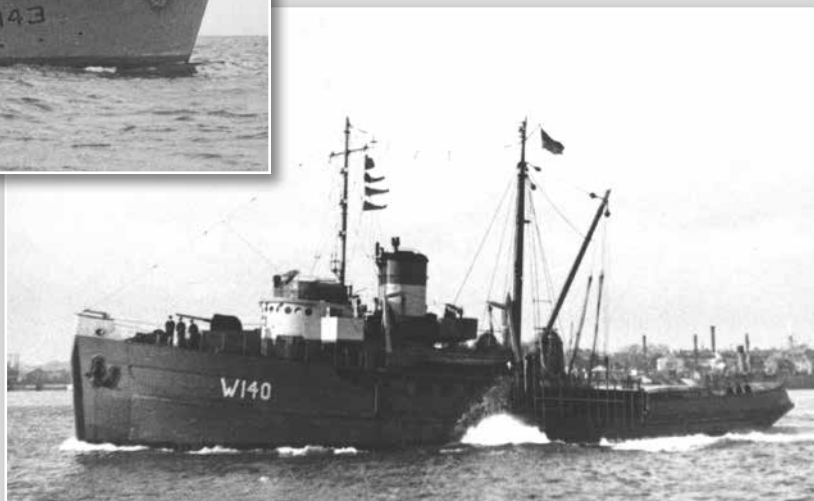
JUSTICE (W 140) - ex BATR 20 - built 1944 Camden Shipyard. - triple expansion 1.875 ihp - 12 knots - wooden hull - later ST. CHRISTOPHER. Armed with 1x 3" AA, 2x 20 mm AA. One of a series of 4 made available under Lend/Lease
