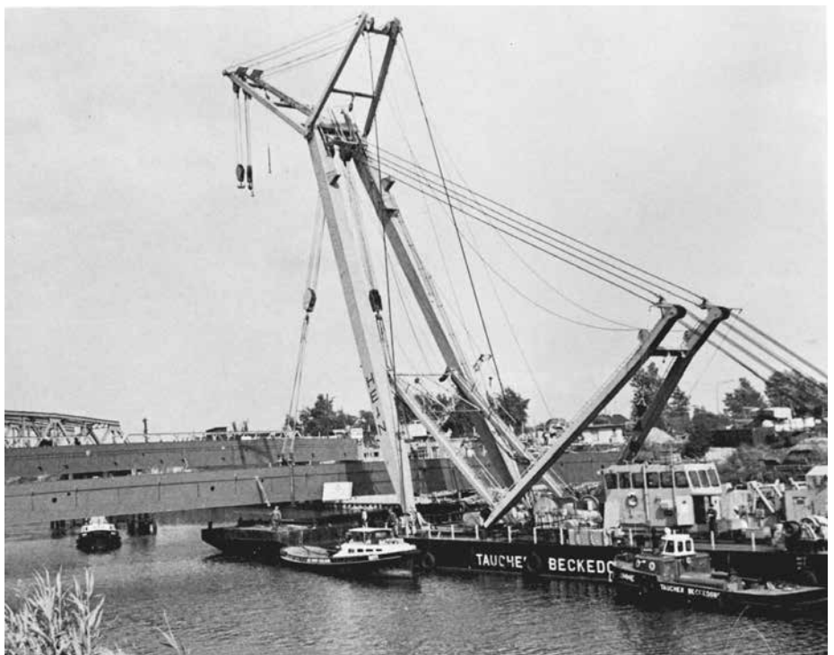
HEIN was built for the Harms associate / subsidiary Beckedorf, better known as Taucher Beckedorf. Seen here installing a bridge span. Alongside aft is the Beckedorf workboat LUMME photo: Ulrich Harms brochure
