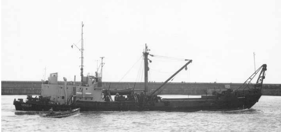
TOPMAST 18 was one of the LCT's acquired by Risdon Beazley and converted for salvage work. TOPMAST 18 was difficult to manoeuvre since her original propulsion had been retained. The fixed-pitch twin propellers both rotated in the same direction. This had come about because of the war construction. The design was such that she had to be able to complete one cross-channel trip to the invasion beaches but otherwise was expendable.
