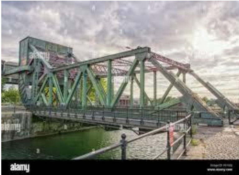
STEEL ROLLING BASCULE BRIDGE
