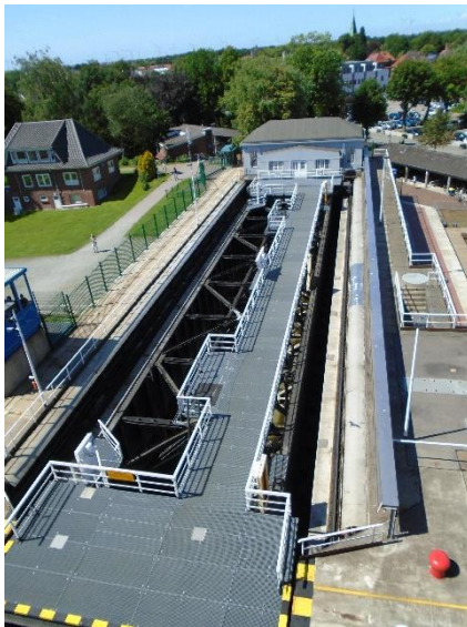
HOLTENAU GATE IN ITS RECESS
