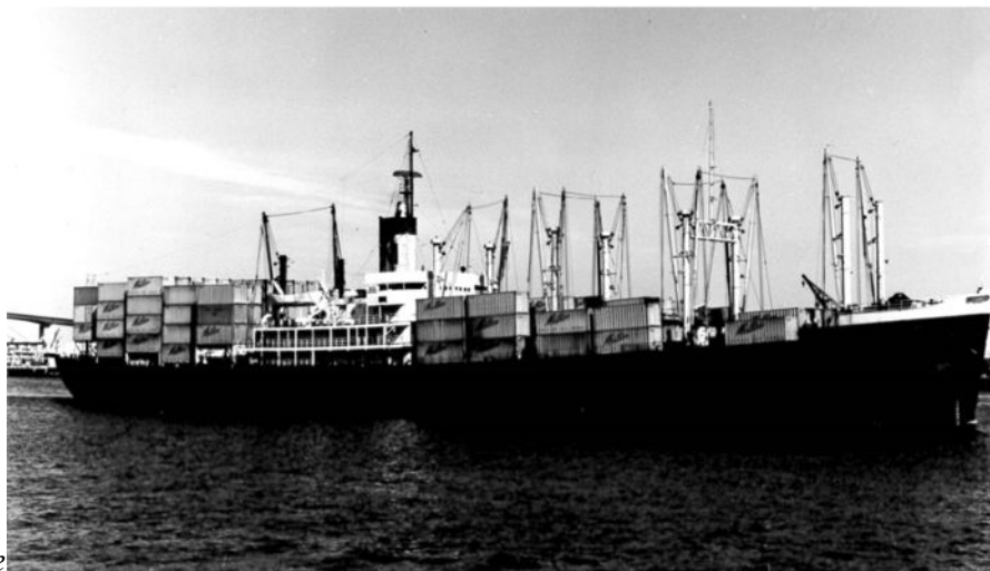
As time passed, the C3s were modified to enable them to carry more containers. In this picture, the Hawaiian Merchant has a substantially larger deck load of containers than the 20 boxes that had been carried on the ship's pioneering voyage to Honolulu on August 31, 1958.
