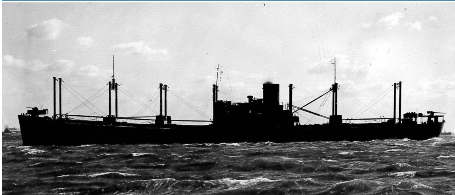
A US Coast Guard photo of the Hawaiian Shipper taken on November 14, 1942, shows the different silhouette the ship presented compared to Matson's standard postwar C3 freighters. The obvious differences include the lower superstructure, shorter stack, and lack of a raised forecastle.
