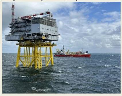
built by Atlantique Offshore Energy, the Chantiers de l'Atlantique division dedicated to marine energy. Foundation installation is underway at the construction site, with the first jacket installed earlier this month. The Dieppe Le Tréport offshore wind farm will feature 62 Siemens Gamesa 8 MW turbines. (Source: Offshore Wind)
