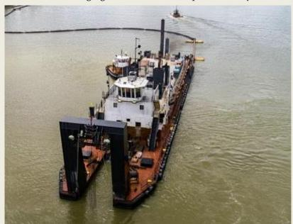
Defense, work consists maintenance dredging approximately 2.7 million cubic yards of sediment within the Delaware River, Philadelphia to Sea main navigation channel (between Stations 117+000 and 237+500). This includes hydraulic dredging with of the dredged placement material into the Pedricktown, Killcohook, Artificial Island and/or Reedy Point disposal areas. The estimated completion date for the project is March 1, 2024. (Source: Dredging Today)
