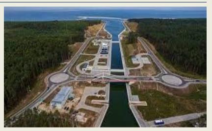
awarded the contract for the construction to the BESIX-NDI joint venture back in 2019. *The works included:* - construction of a navigation channel through the peninsula, two breakwaters of respectively 1,014 m and 568 m long, - two rotating steel bridges with lock infrastructure, - sluice gates, buildings and a new road system. On top of that, a 180 ha artificial island was created with the excavated earth, which will now serve as a protected shelter for birds. The navigation channel is 1.3
