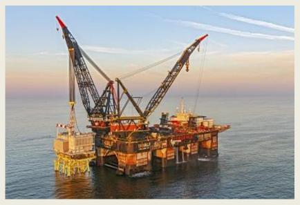
With the help of the crane Thialf. vessel the superstructure (topside) for the offshore transformer platform Hollandse Kust (west Alpha) has been successfully placed on the undercarriage (jacket). This milestone for new the connection of offshore wind took place last night about 50 kilometers off the coast of Egmond aan Zee. From 2026, grid operator TenneT will bring sustainable wind energy onshore via this 'socket'. The
