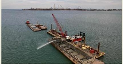
channels so freighters can reach the coal docks. The dredged material is then pumped to the new wetlands facility for safe storage and to create new bio-friendly wetlands. *(Source: Dredging Today)*
