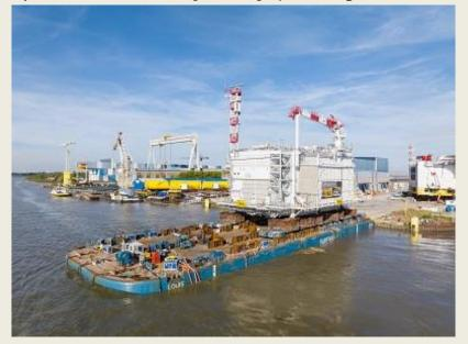
vessel **Orion**, the topside of 47 metres long, 35 metres wide and 25 metres high will be placed on the undercarriage and then welded in place." *First delivery* Two years after the first steel cut, the topside, built by the EQUANS/Smulders
