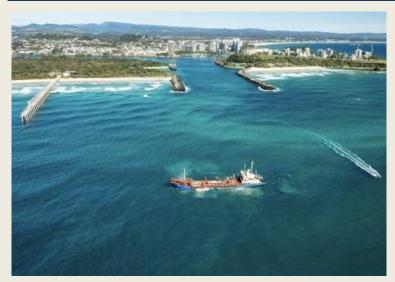
Transport for New South Wales (TfNSW) is currently seeking to suitably qualified engage organization undertake to maintenance dredging of the Tweed River Entrance. Despite the jetty that collects most of the coastal sand drift, some sand still moves past the jetty and into the Tweed River entrance. This sand builds up over time, requiring periodic dredging. The sand is removed from the Tweed River entrance and deposited to locations offshore. Keeping the
