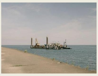
Sodus Bay, the contractor first completed dredging work in Oak Orchard Harbor, where approximately 15,000 cubic yards of material was dredged from the federal navigation channel and placed in designated open lake sites. Dredging of both harbours is conducted by USACE on an infrequent basis, based on need and the availability of funding. Oak Orchard Harbor was last
