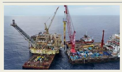
Malaysia's largest offshore removal project now part of rigto-reef marine habitat. Marine Masters has successfully completed its offshore scope for the decommissioning of the South Angsi Alpha (SAA) platform, operated by Hibiscus Oil & Gas Malaysia Limited. The campaign marks a major milestone in the repurposing of retired offshore infrastructure,
