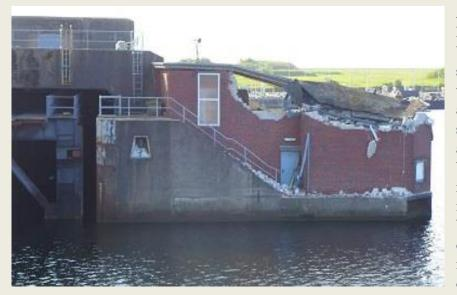
A naval vessel rammed the lock in gate Wilhelmshaven, causing significant damage. wheelhouse was destroyed, and debris had to be salvaged. The cause of the accident remains unclear. Wilhelmshaven - The task force supply ship "Berlin" rammed the lock head between the two chambers of the fourth entrance with its bow on Sunday evening, causing significant damage.
