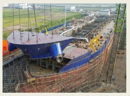
ZPMC said today that a major milestone has been reached in of construction new  $30,000 \text{m}^3$ trailing suction hopper dredger (TSHD), as the vessel's main hull has been successfully completed. This achievement lays a solid foundation for the next phase of equipment installation and commissioning, the company said. The new giant dredger combines advanced capabilities such as ultra-deep dredging, powerful cutting, and long-distance
