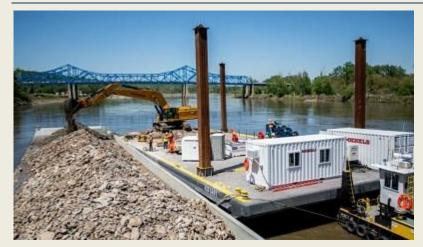
Work is well underway on the USACE Omaha District's bedrock removal project in the Florence Bend reach portion of the Missouri River near Omaha. The implementation of the excavation is due to riverbed degradation in recent years, which has lowered water elevation at certain river stages through this reach of the river. This has resulted in insufficient navigation channel
