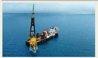
Heerema Marine Contractors' heavy lift vessel Aegir has completed the installation of jacket foundations at the Greater Changhua 2a wind farm site offshore Taiwan and will now move on to do the same work on Greater Changhua 1, the company said via social media. This brought the entire 900 MW Greater Changhua 1 & 2a project to having around half of the jacket
