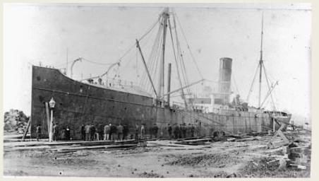
SS Hilonian was a general passenger and cargo steamer. built the as **Triumph** 1880 in at Middlesbrough for McIntyre & Co, and later fitted with refrigeration equipment and leased to Shaw Savill and the New Zealand Shipping Company. She sank and ran aground many times, the final sinking being
