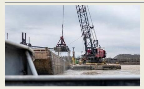
The U.S. Army Corps of Engineers Buffalo District's first dredging project of the year has already wrapped up – ahead of schedule. USACE moved over 80,000 cubic yards of dredged Lorain material from Harbor to provide ease of navigation and passage for large vessels carrying products vital to the economy. Dredging in Lorain occurs once every 3
