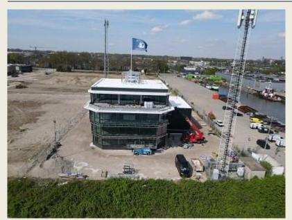
Tug and workboat company Herman Senior are excited to share the latest update on the construction of their new office and warehouse. The glass has now been fully installed, and all interior flooring is completeboth in the office spaces and the warehouse. On the exterior, insulation has been placed and panelling has begun. Everything is progressing according to plan, and if all continues to run smoothly, they expect delivery in July 2025. From that point, they will focus on the final
