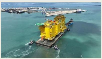
**Pioneering Spirit**, according to Dragados Offshore. After the transfer of both jacket and topside, it will continue its journey to the installation site in the German North Sea. The total transport time is expected to take approximately two weeks, and the installation offshore another two weeks, said the
