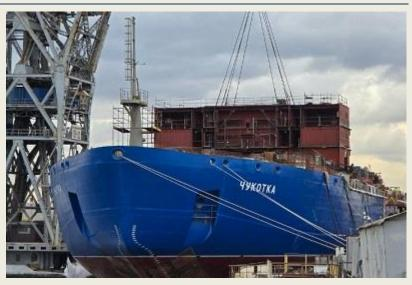
width is almost 12 m. After installation and assembly, the block will continue to be equipped and the arrangement of the interior will begin. The superstructure of the icebreaker, which includes the installed block, will house the wheelhouse, cabins for the crew, recreation areas, sanitary and
