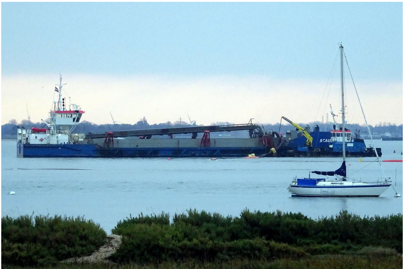
Recharging beaches and other sites with dredged spoil is being carried out at four sites around Mersea Island. Here “ Scald ” is seen attaching the pipeline assisted by “ MCS Anneke ” to recharge Cobmarsh Island in West Mersea harbour on 21 st December. (Photo by Ian Clarke)
